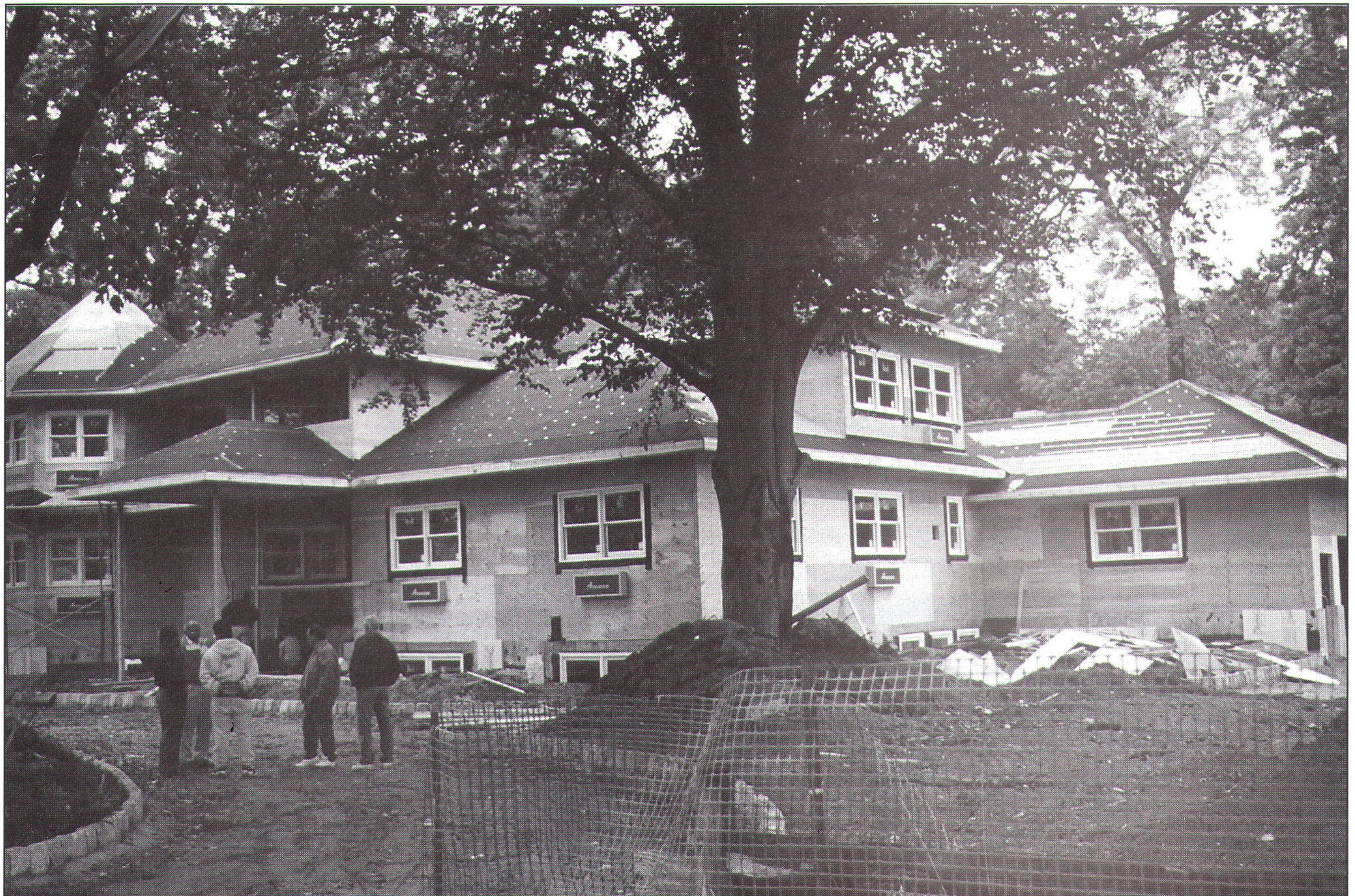
Diocesan Center work in progress: Picture taken in October, 1997
