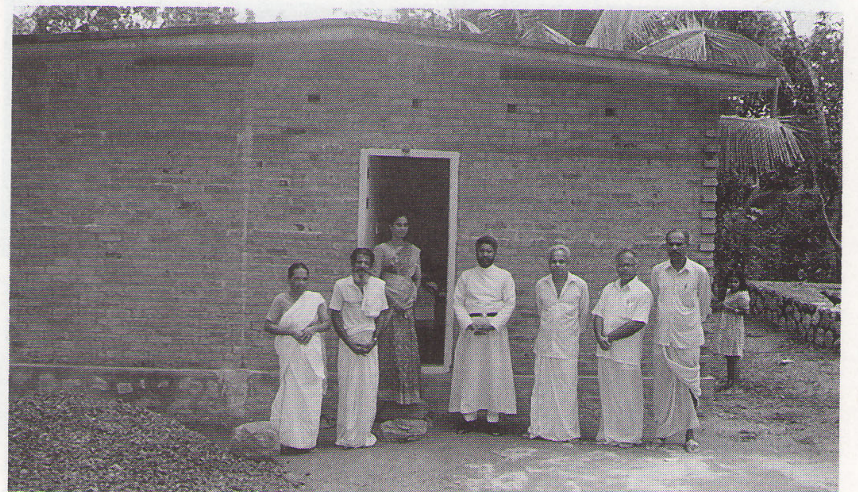
Another house being completed
